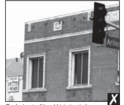
Replacing traditional historic windows with aluminum sliding windows like these is inappropriate.
