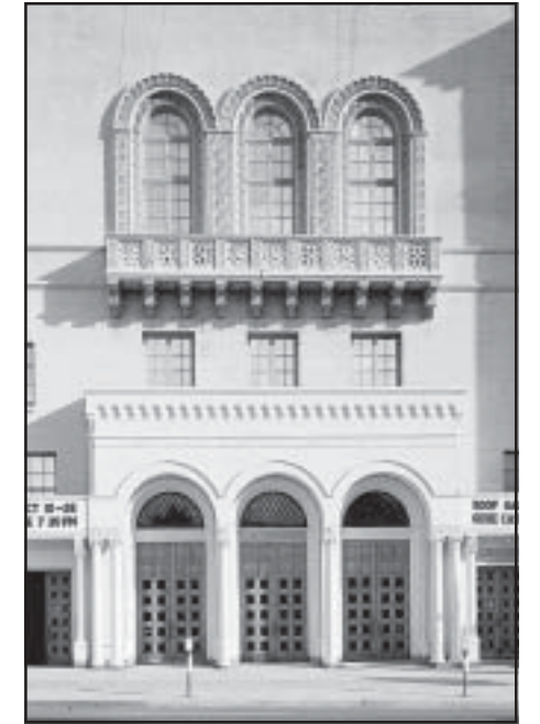
These windows have a heavily decorative surround which echoes their arched form.
