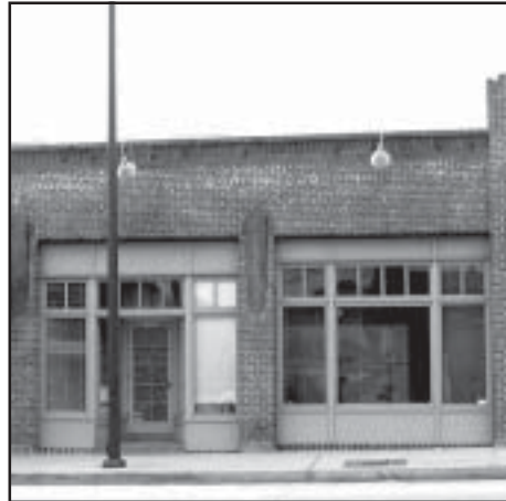
A simple, unornamented two-bay storefront.
