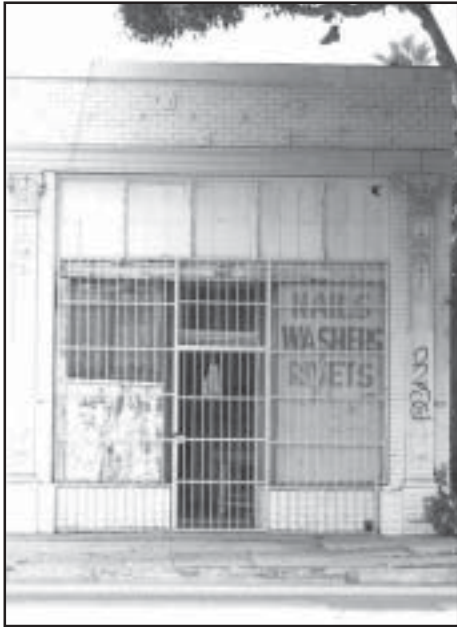
Fixed bars like these are inappropriate on historic storefronts.
