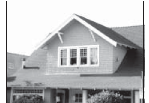
Second story dormer roof element
