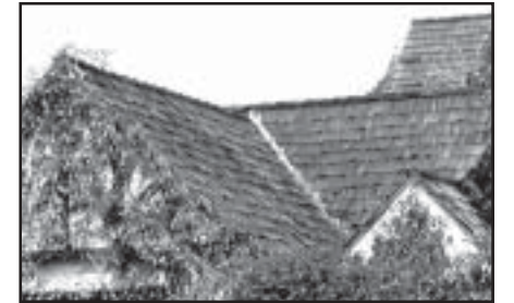
Wood shingle roof
