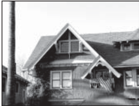
Complex multi-gabled roof with composition shingle
