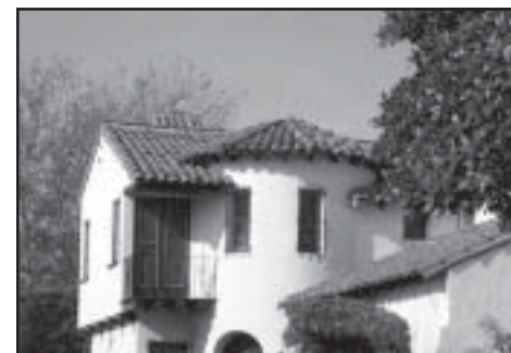
Complex roof plan with terra-cotta tile
