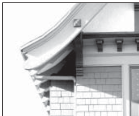
Decorative rafter tails help define this house
