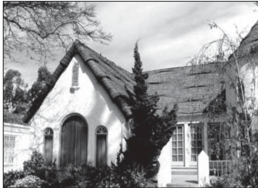
Built-up faux thatch shingle roof
