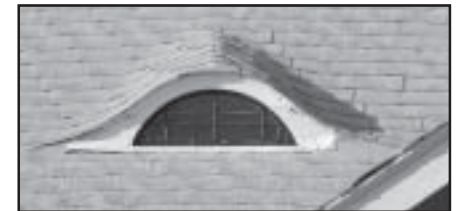
Composition shingle roof with an eyebrow dormer
