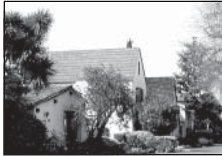
Tile, slate, and wood roofs
