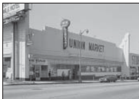
Others had flat roofs with decorative parapet detail, like this art deco market.
