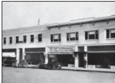
Cornice details help distinguish commercial buildings.
