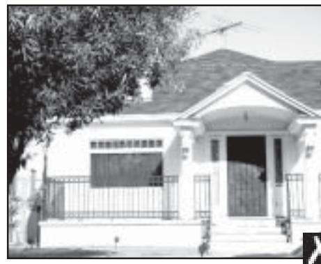
The added iron balustrade is inappropriate on this porch.
