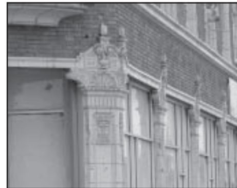
Glazed terra cotta tile detail was common in the early twentieth century on commercial buildings.
