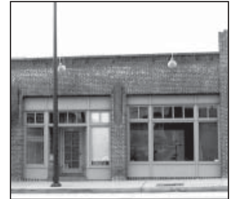
Simple brickwork was a common feature on early twentieth century commercial buildings.
