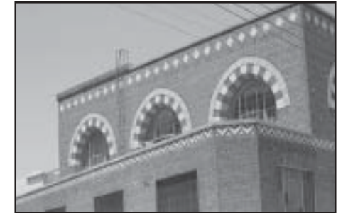
Architectural detail in commercial buildings can be applied, or can come from the contrast of materials.
