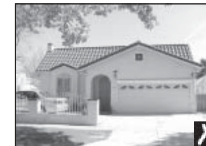
This front-yard garage is out of place in most historic contexts.
