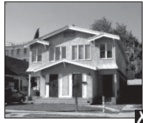
Stucco has completely concealed the original building materials of this house.
