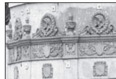
Applied detail on smooth stucco.
