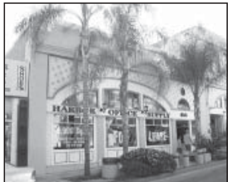
Tile detail adds character to this structure.
