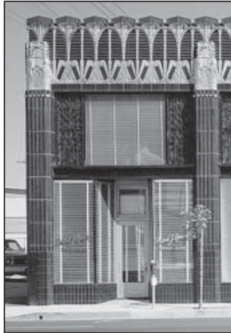
Terracotta and gilded detail were hallmarks of the art deco style.
