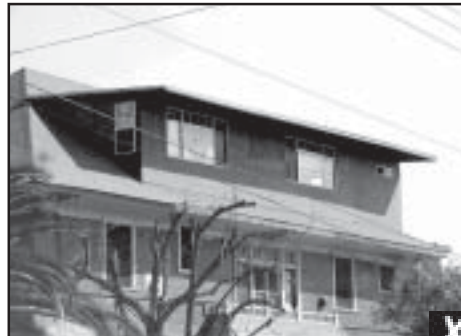
Inappropriate rooftop addition located on a street-facing facade with incompatible windows
