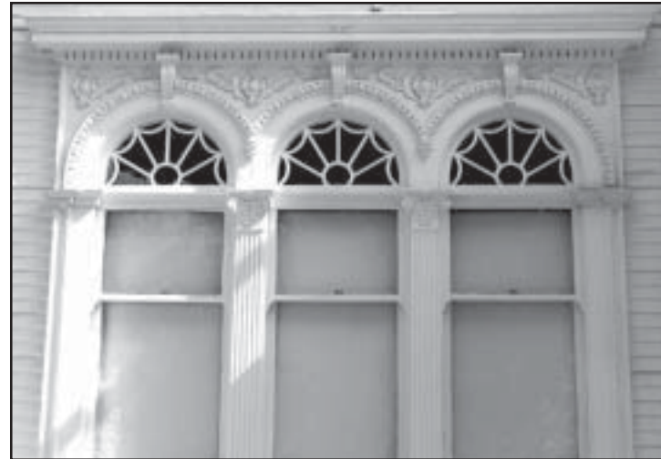
Triple double-hung one-over-one wood windows with decorative fan lights
