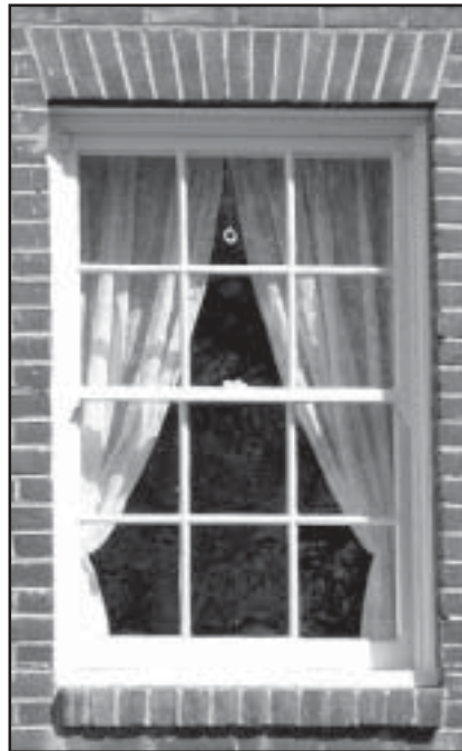
Six over six wood double-hung window
