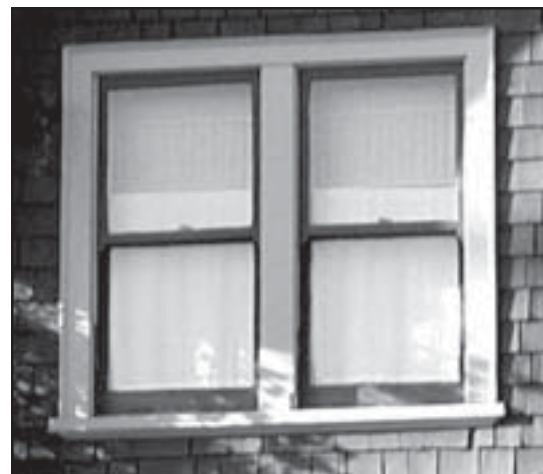
Paired double-hung wood windows
