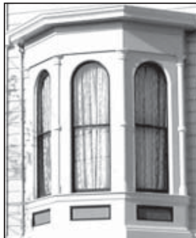
Rounded-top double-hung wood bay windows
