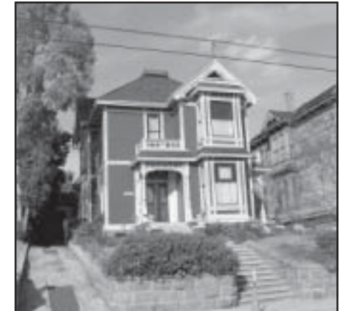
Historic stone retaining walls and steps.
