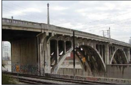
A view of the current Spring Street Bridge
